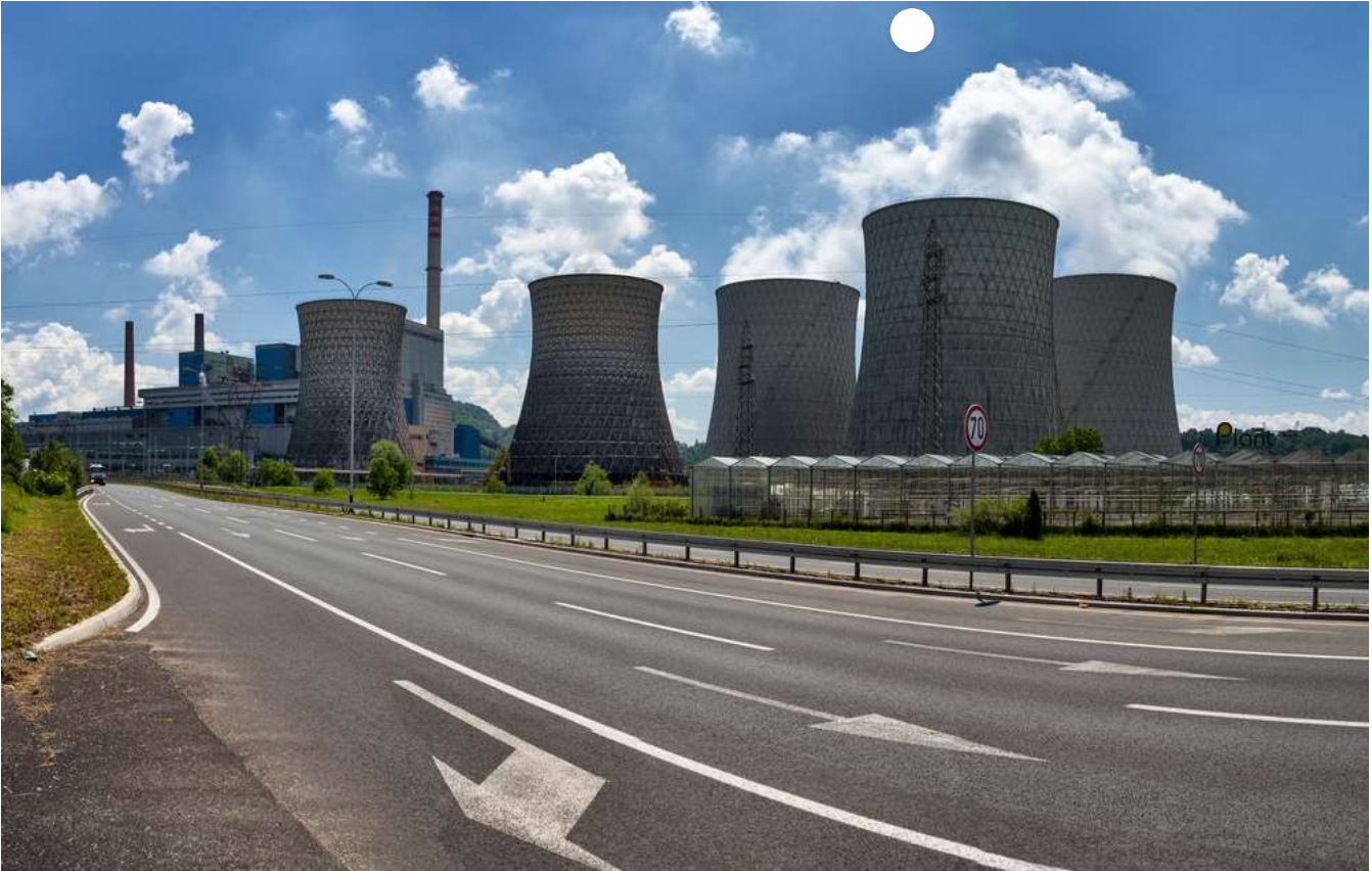
Tuzla, la centrale termoelettrica © goodcat/Shutterstock
